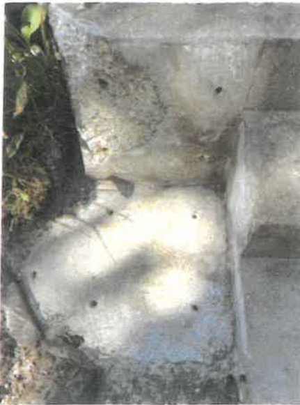
Left footing with dowel holes
