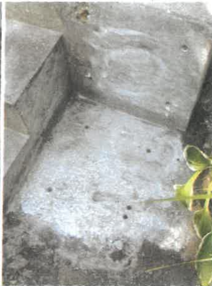
Right footing with dowel holes
