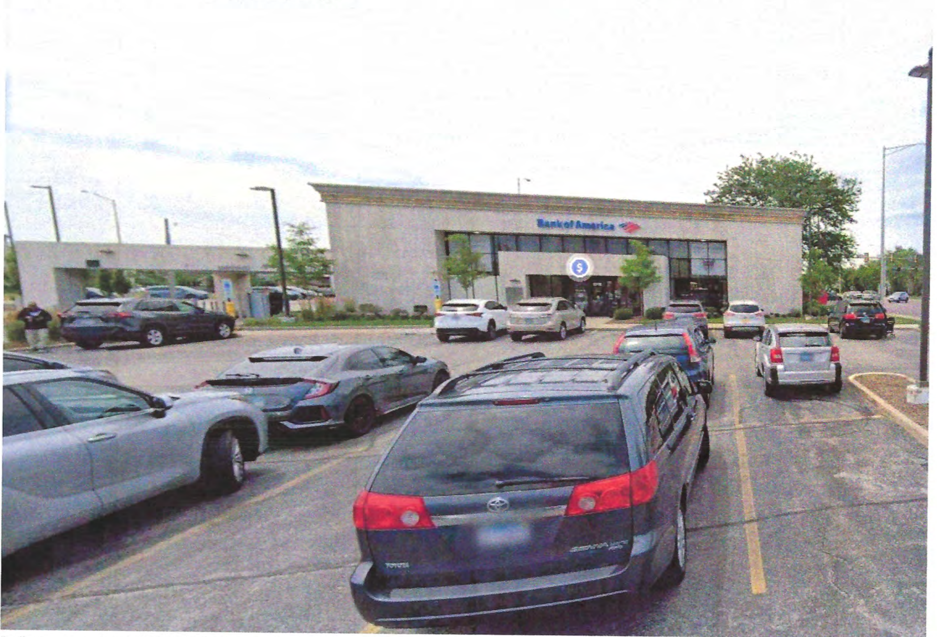
East elevation entrance view from parking lot
