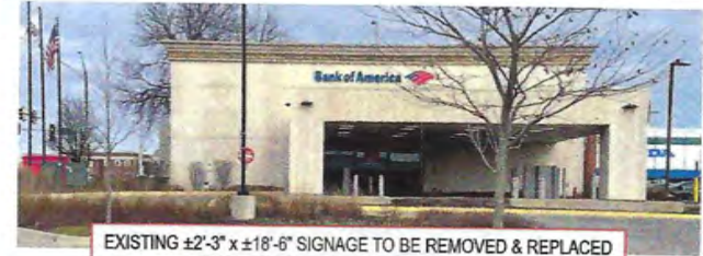
EXISTING ±2'-3" x ±18'-6" SIGNAGE TO BE REMOVED & REPLACED WALL TO BE PATCHED & PAINTED BY GC
