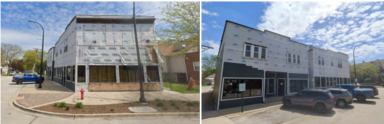
Existing Cornice (LEFT); Partially Installed Hardie Board (RIGHT)
