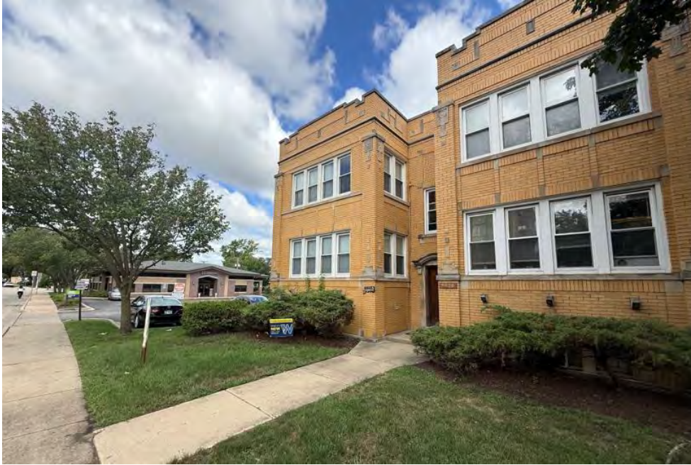
Photos of Subject Property (5926-28 Lincoln Avenue) and adjacent building (5940 Lincoln Avenue)
