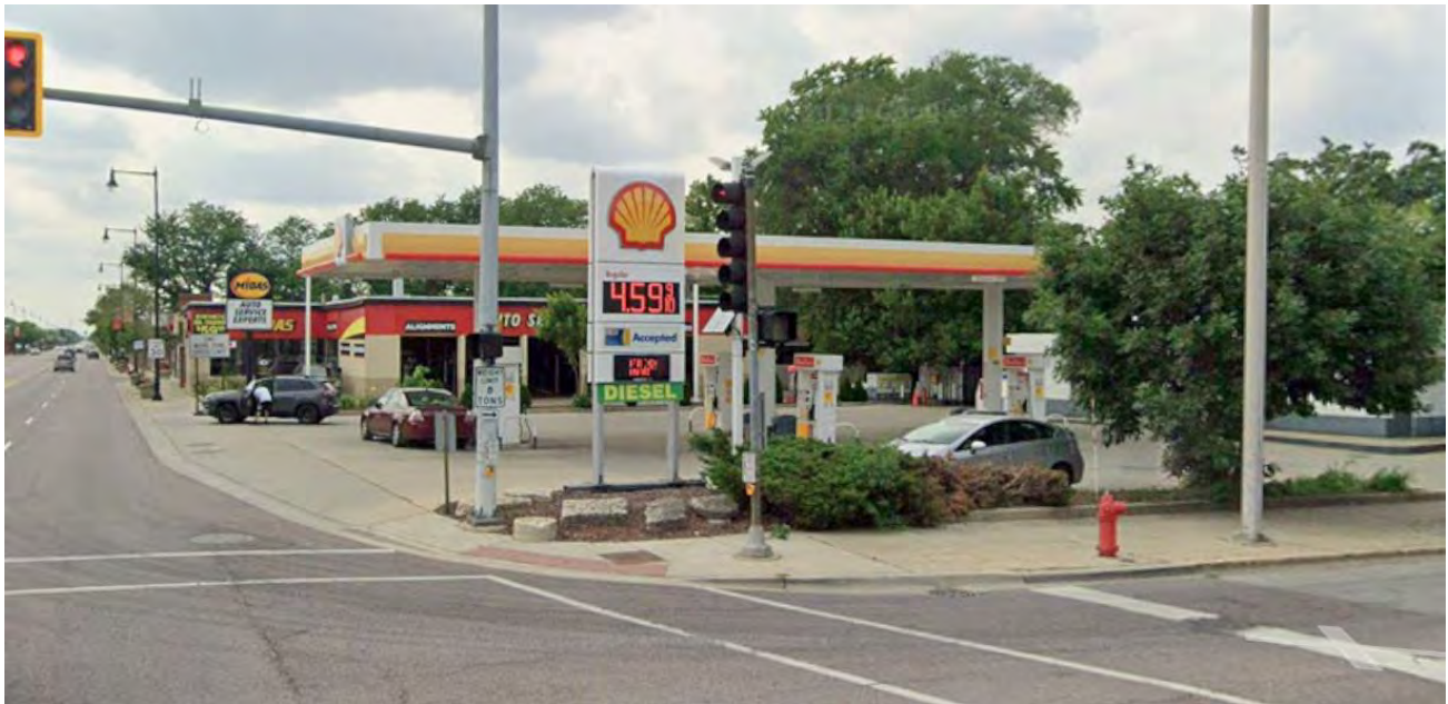
Existing Pole Sign at 5600 Dempster Street
