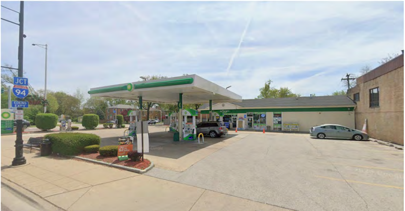
BP Station at 5601 Dempster Street
