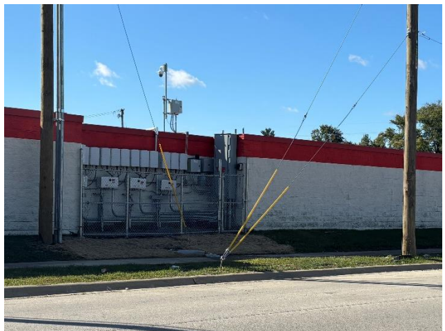
Roof-mounted Solar Energy Collection System with Façade-mounted Inverter Racks protected by a Chain Link Fence (Public Storage, Chicago Heights, IL)
