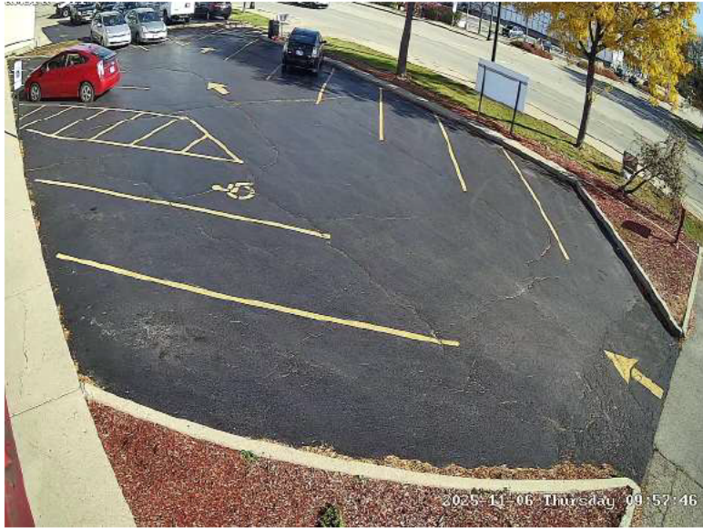
Looking north at Parking Lot
