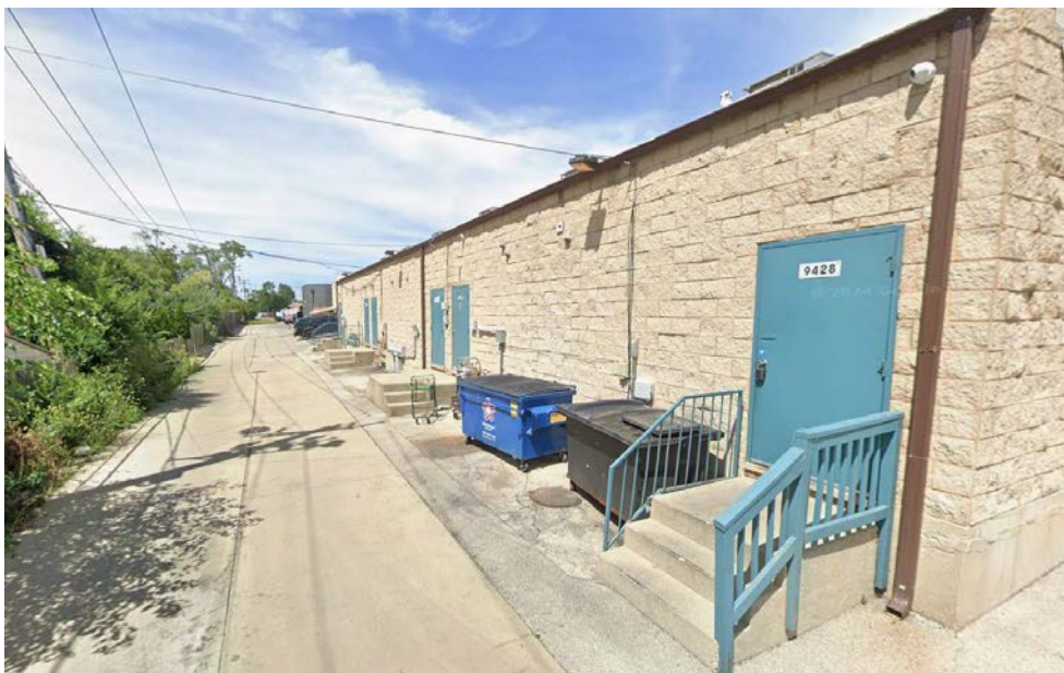
Rear Alley at Subject Property where parking has been Observed
