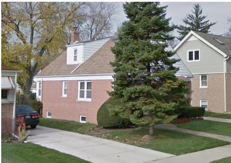
Subject Property Street View Showing Existing Basement Window
